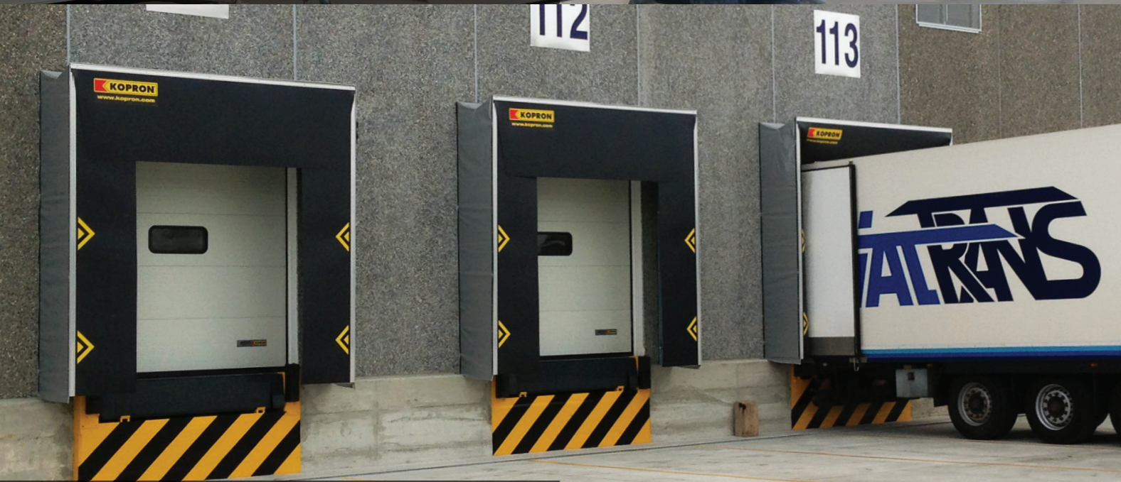
BERGAMO (BG) - ITALTRANS - WAREHOUSING, HANDLING AND DELIVERY
